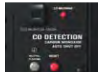
Carbon Monoxide Detection & Auto Shut Off
